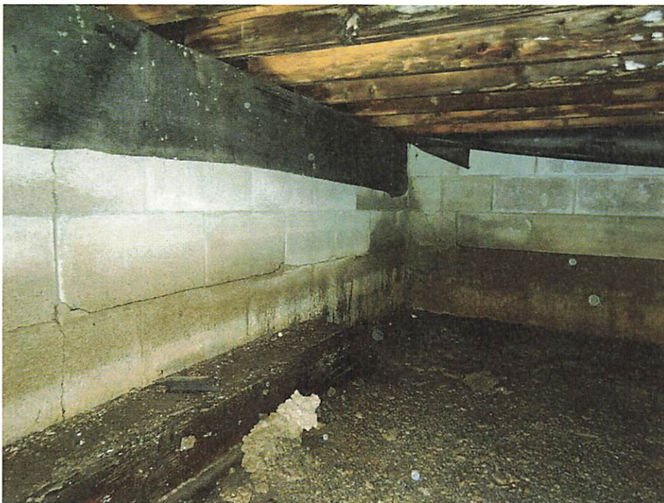
Photo 22. Crawlspace under addition looking west
