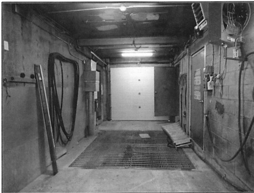
Photo 26: Zamboni Room looking East
