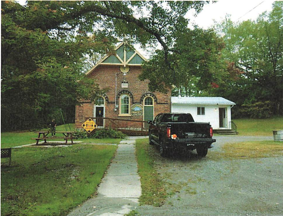
Photo 1. Building north elevation (front)
