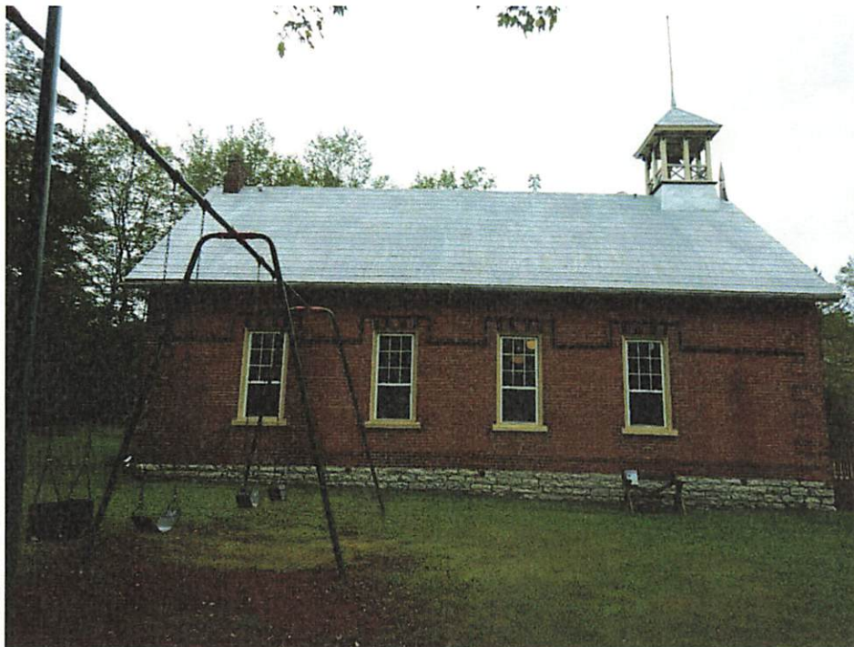
Photo 4. Building east elevation
