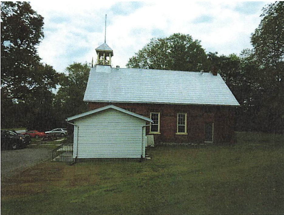
Photo 2. Building west elevation
