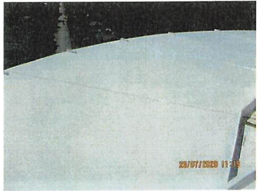
Another random view of tank roof plating
