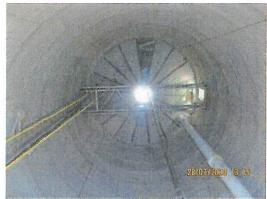
Overall view – looking up - of concrete structure
