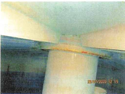
Underside of roof structure viewed from manway
