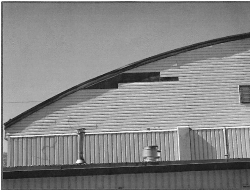
Photo 10: Removed Siding on East Elevation
