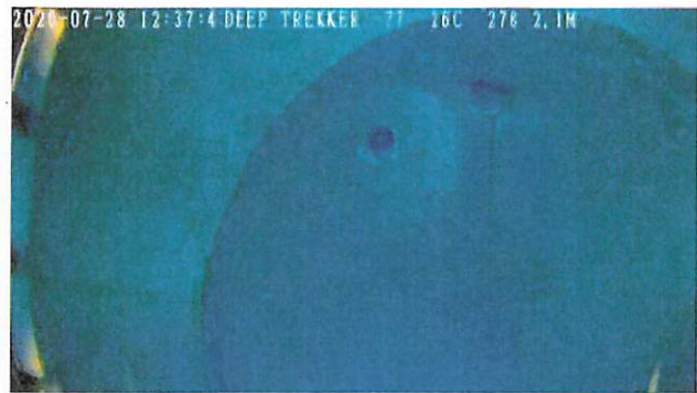
Straight down, wide view of tank floor
