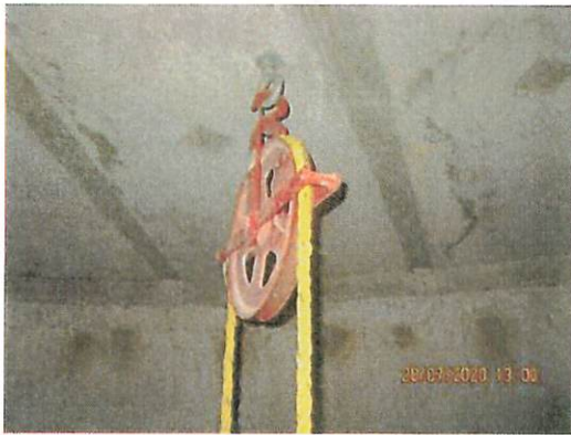
Pulley used for hoisting equipment to tank catwalk
