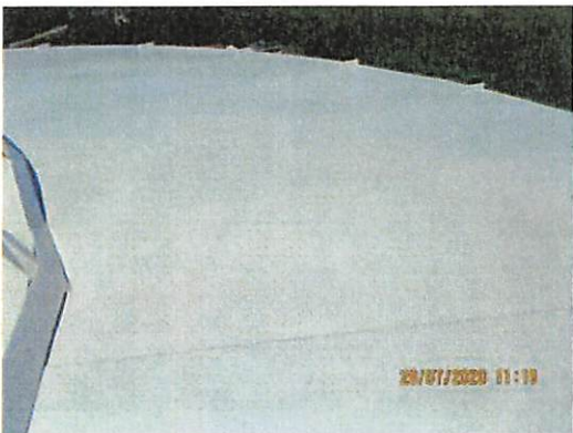
Random section of tank roof; coating in good condition
