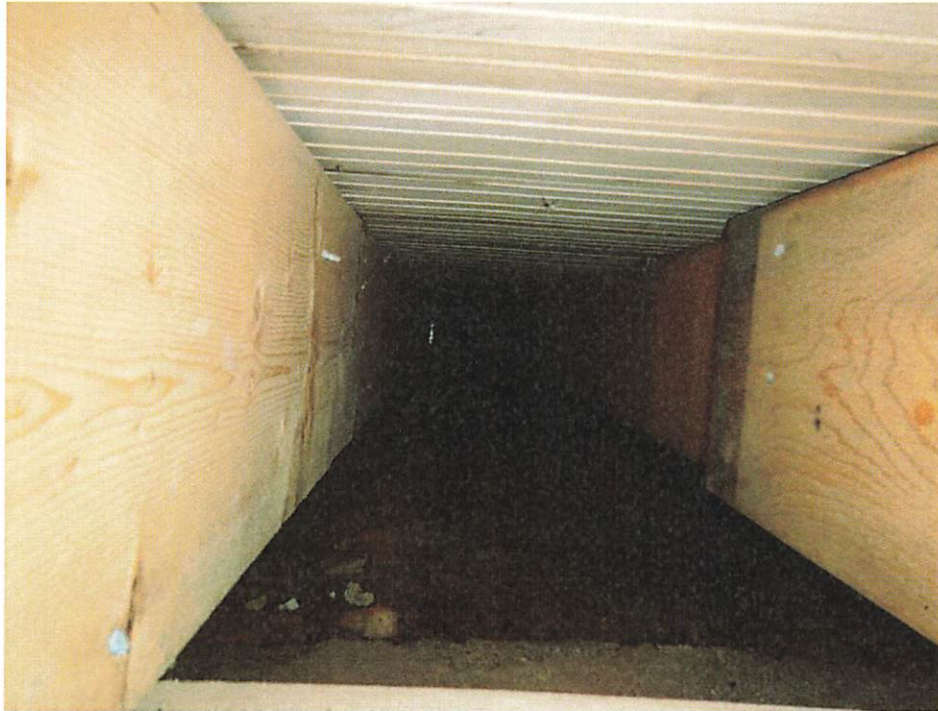
Photo 19. Crawlspace on south side of original building
