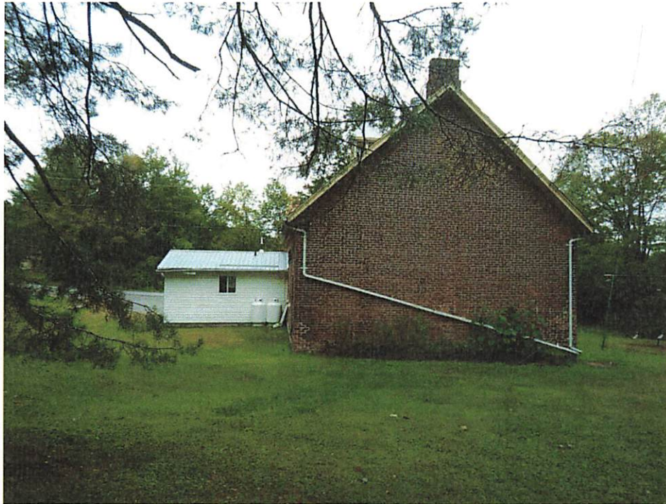
Photo 3. Building south elevation (rear)
