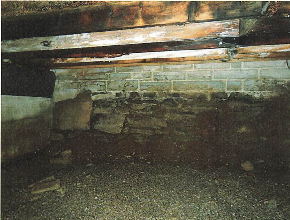
Photo 23. Crawlspace under addition showing connection to original structure
