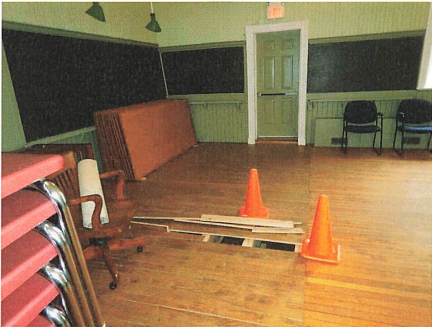
Photo 13. Removed floorboards on south side of building
