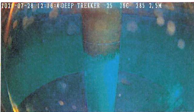
Staining on dry riser at water level fluctuation zone
