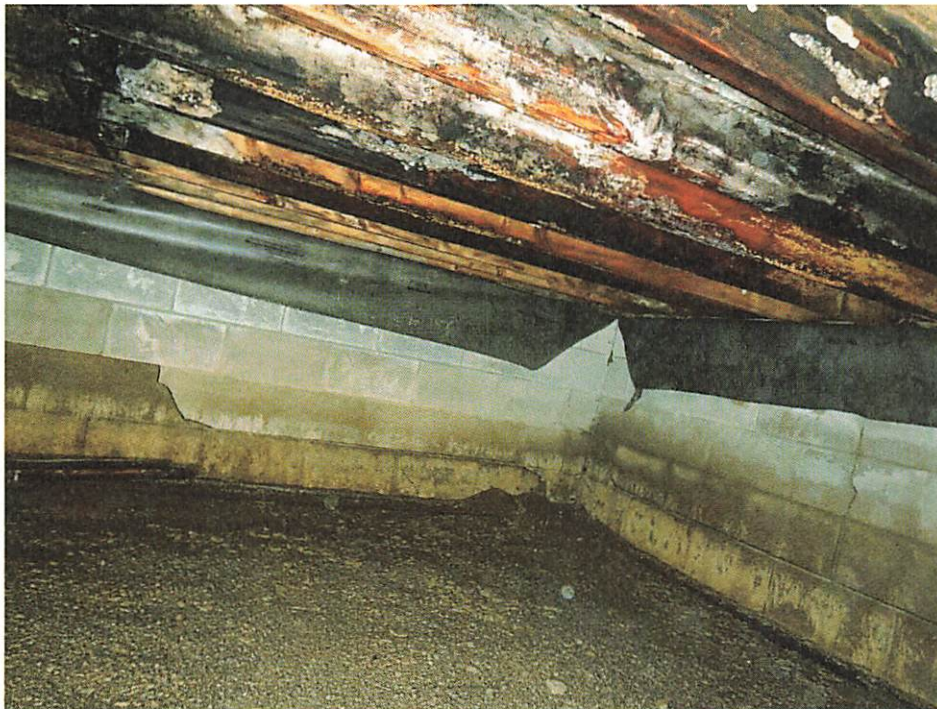
Photo 24. Crawlspace under addition showing condition of floor joists
