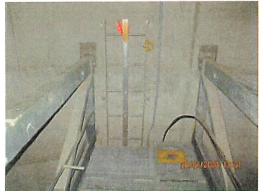
Top end of ground to catwalk ladder
