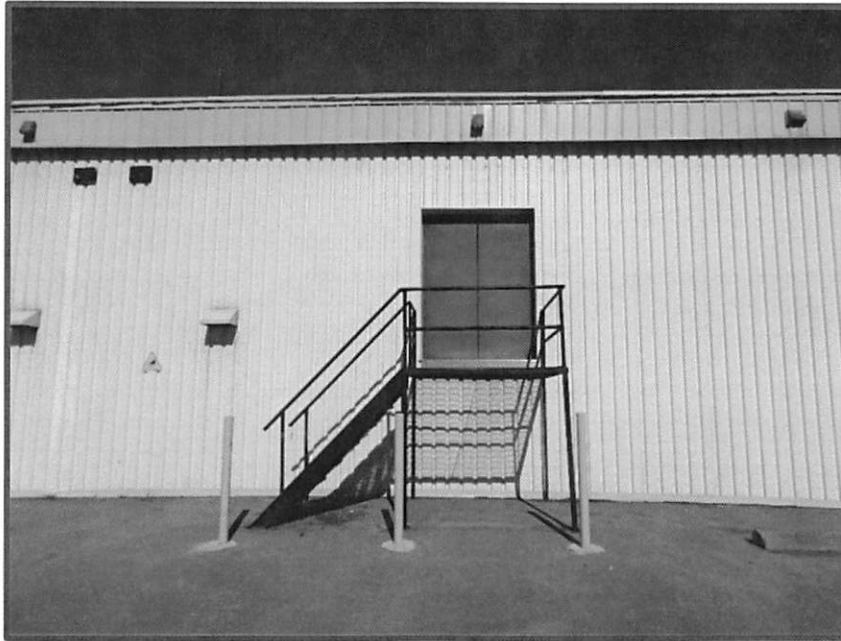
Photo 5: Typical Exit Staircase on South Elevation
