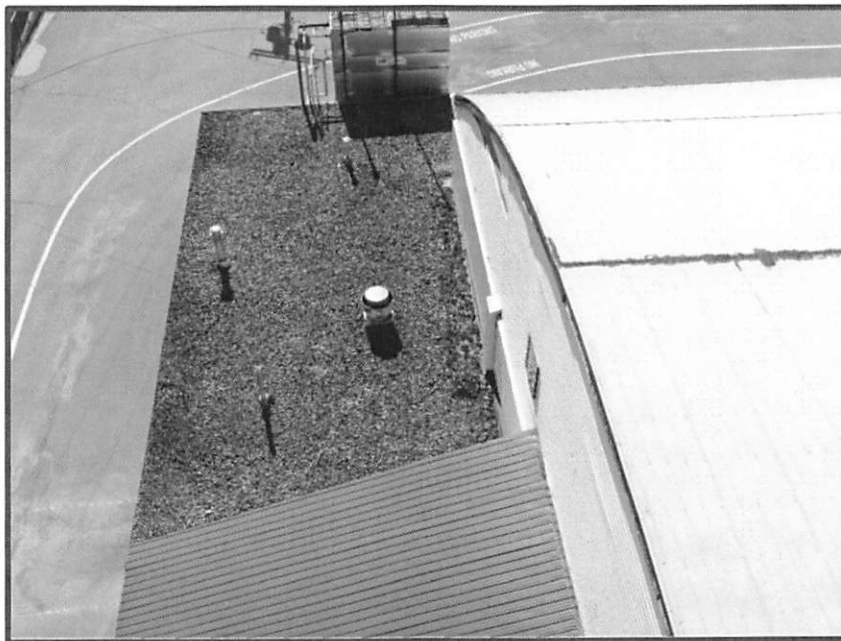
Photo 20: Lower East Roof
