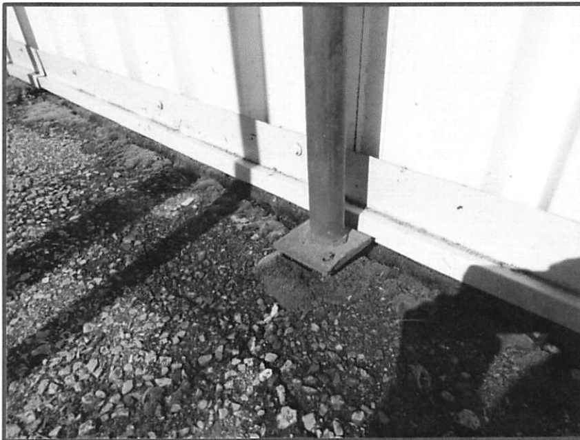
Photo 6: Typical Staircase Support Connection
