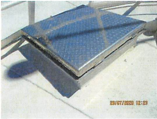
Tank roof hatch closed and secured after survey
