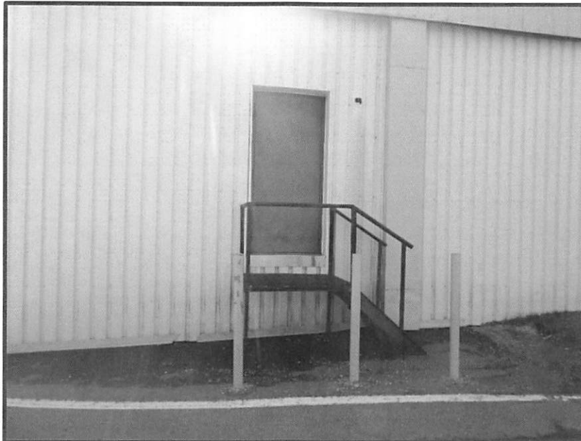
Photo 7: Exit Staircase on North Elevation
