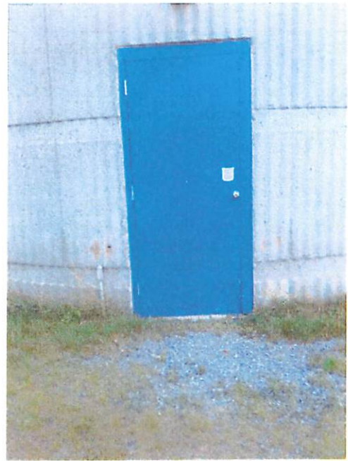
Tower skirt entry door secured after survey
