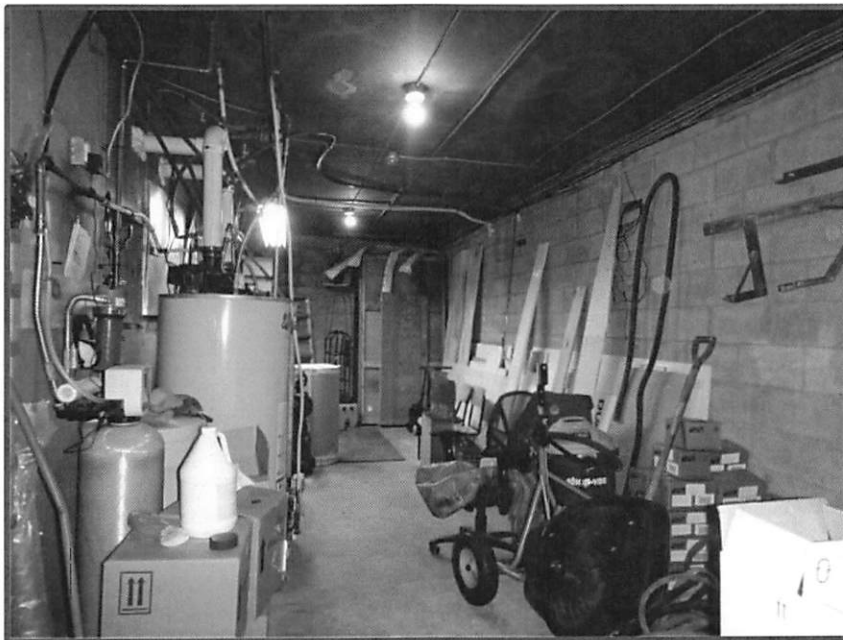
Photo 24: East Storage Room
