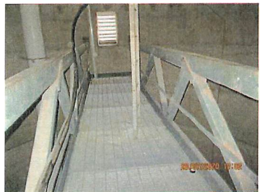
Catwalk and bottom of roof access ladder
