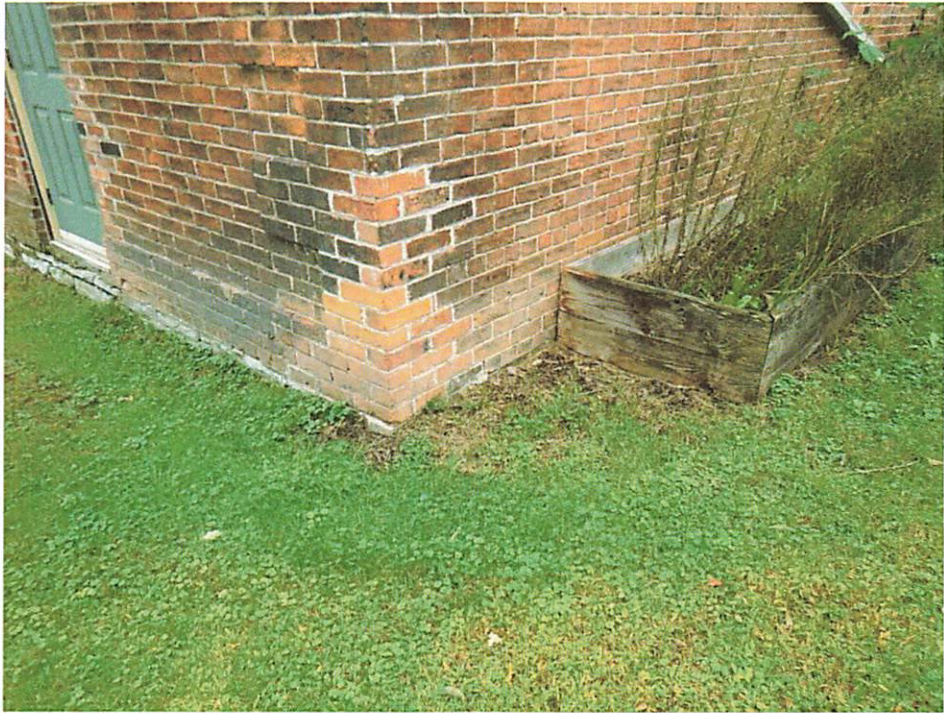
Photo 9. Grading above foundation line
