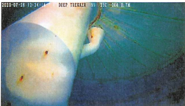
View up dry riser and attached overflow opening
