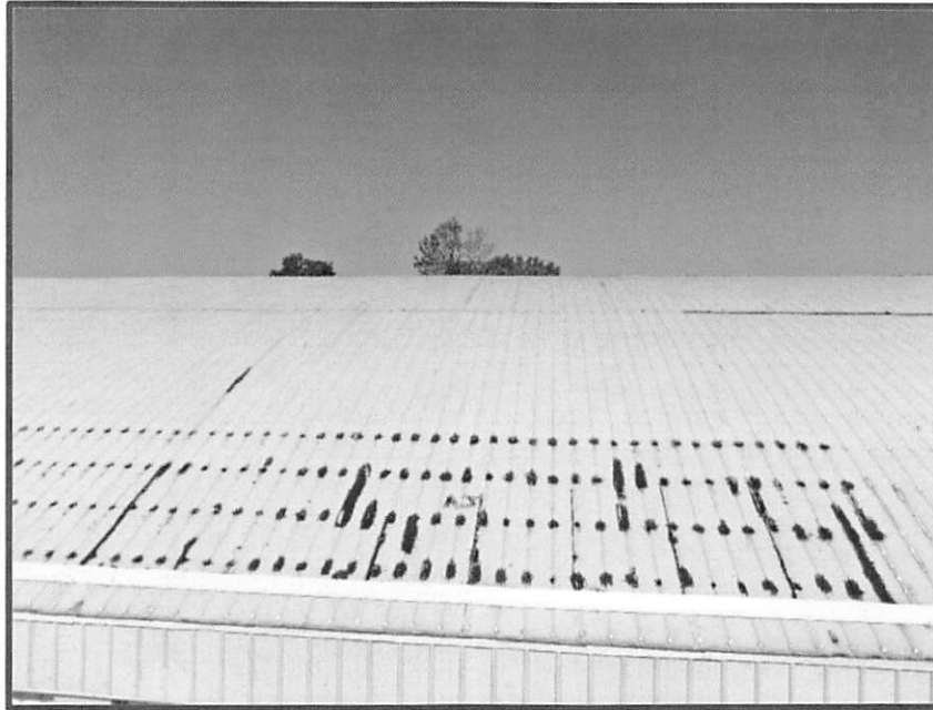
Photo 19: Roof Patching
