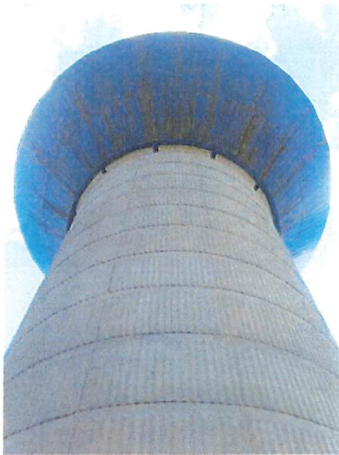
Residue and "growth" deposits under angled section
