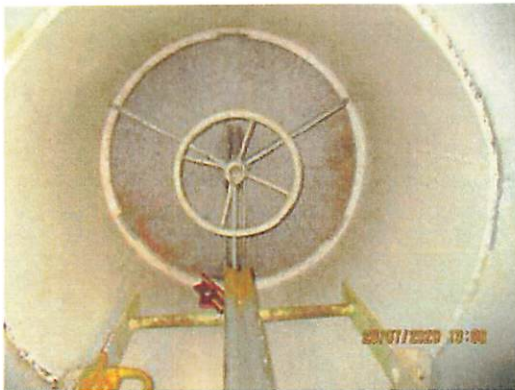
Underside of tank floor hatch
