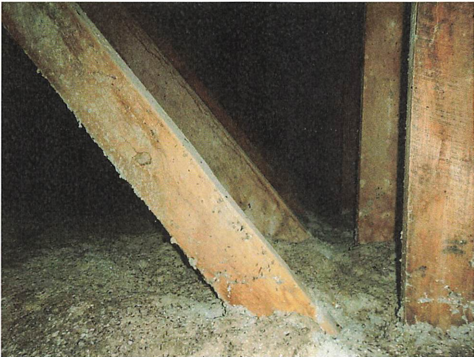
Photo 18. Upper attic space of original building in good condition
