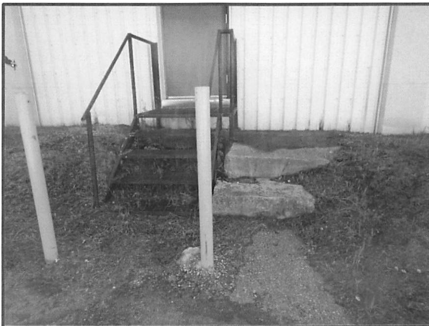
Photo 8: Exit staircase on North Elevation
