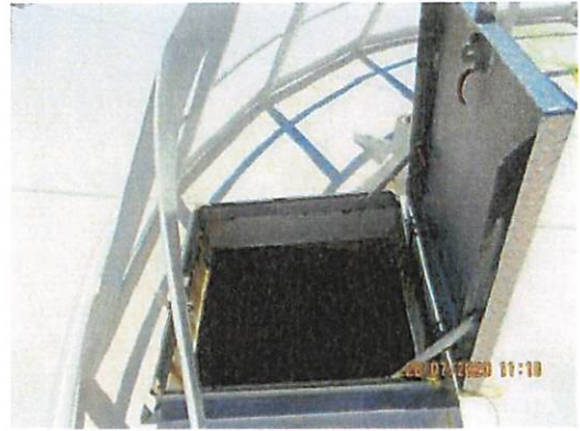
Tank roof hatch opened to allow ROV access
